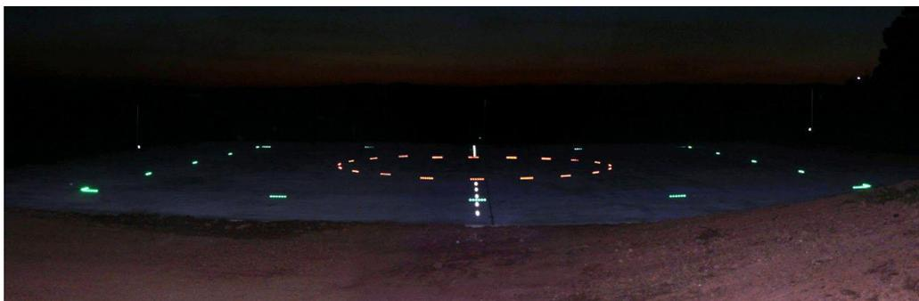
There is a preference to have pilot activated lighting (PAL) with manual backup and linked into the uninterrupted power supply system.
